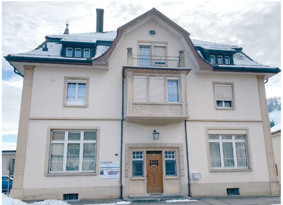
Erker Hulfteggstrasse 5, Gähwil
